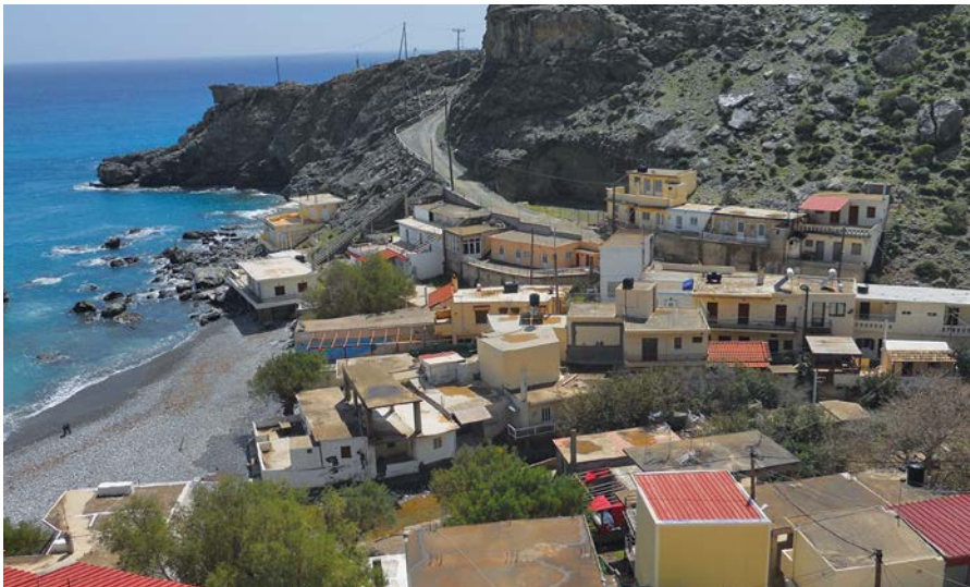
Unregulated building on the coastal zone.
